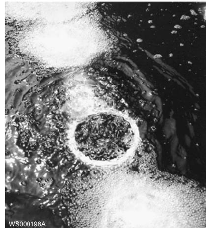
Figure 28: Excessive air discharge
