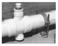
Figure 18: Sump between air distributor sections
